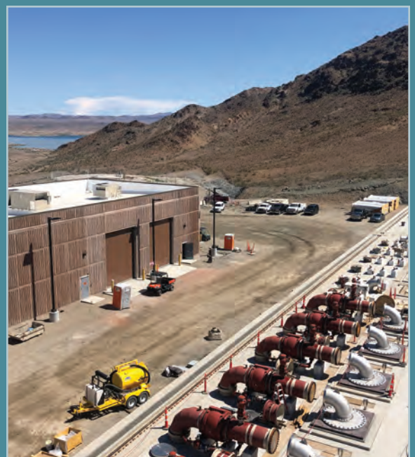
Low Lake Level Pumping Station Construction
